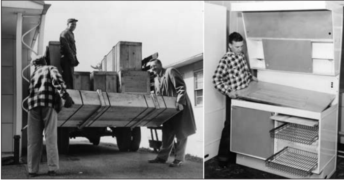
FIG. 12 Shipping and installing the field kitchens, 1954. (left) The demountable units were shipped flat in crates; (right) assembly of mix center at the Housing Research Center Laboratory. (Source: CHES, Box 11, folder 18.)
