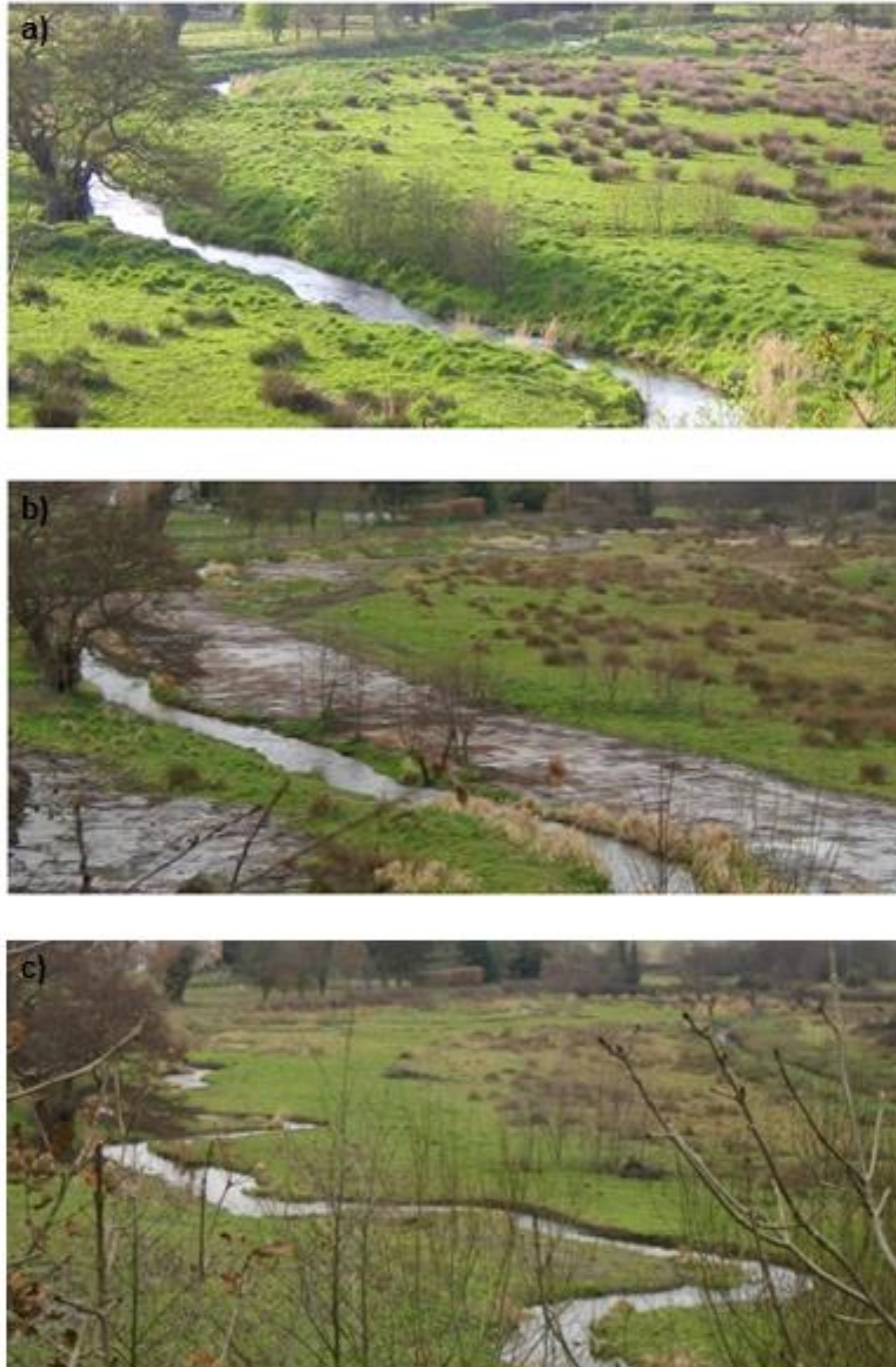
Figure 10.2: Photographs of the River Glaven at Hunworth Meadow showing (a) the river embankments in January 2009 prior to embankment removal, (b) the completed Stage I restoration work with embankments removed in March 2009, and (c) completed Stage II restoration work with embankments removed and remeandered river channel in December 2010.
