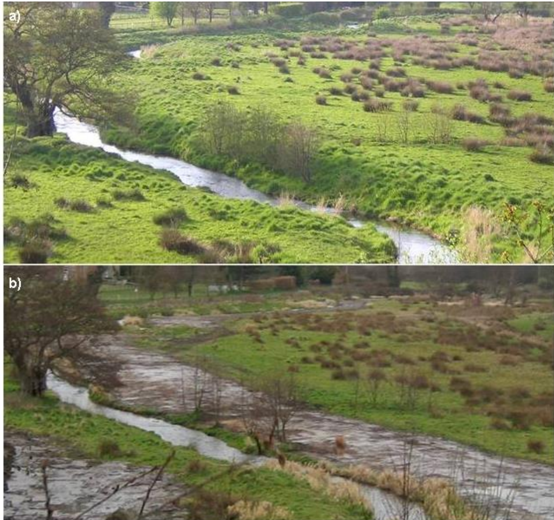
Figure 3.13: Photographs of the River Glaven at Hunworth Meadow showing (a) the river embankments in January 2009 prior to the restoration and (b) the completed restoration work with embankments removed in March 2009.
