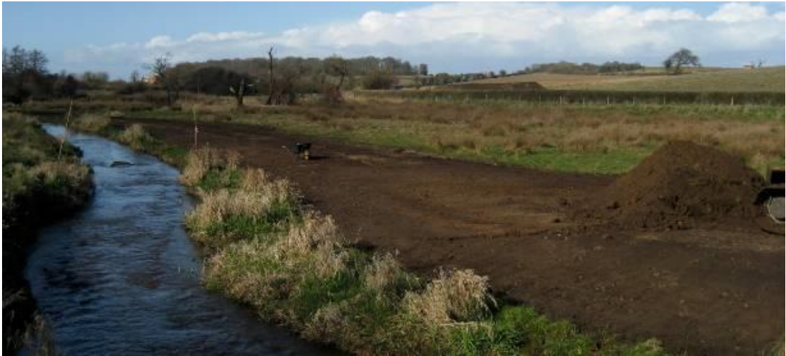
Figure 3.12: Embankment removal work in progress (March 2009).
