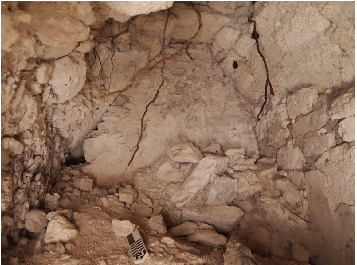
Figure 242 Photograph of Lot 40 fill beneath vaulted roof, Str. TM-2-R2
