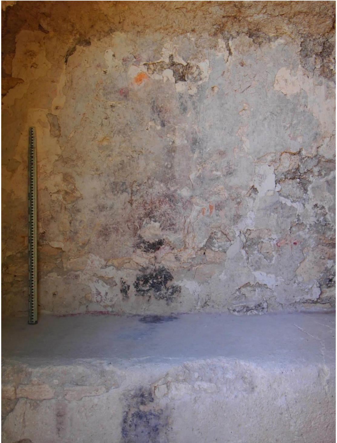
Figure 250 Photograph of overview of painted wall, Str. TM-2-R2
