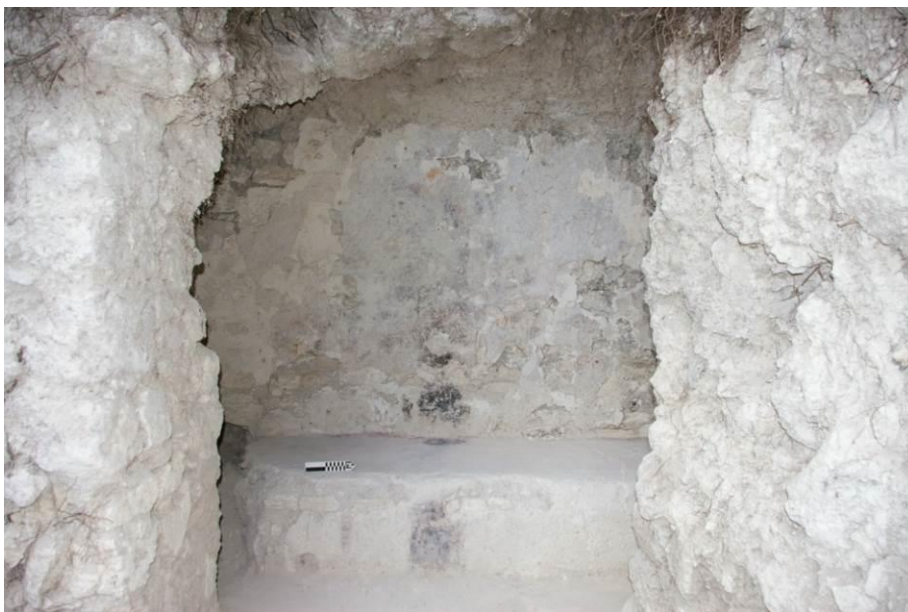
Figure 239 Photograph of burnt area on front of bench, and burning on wall , Str. TM-2
