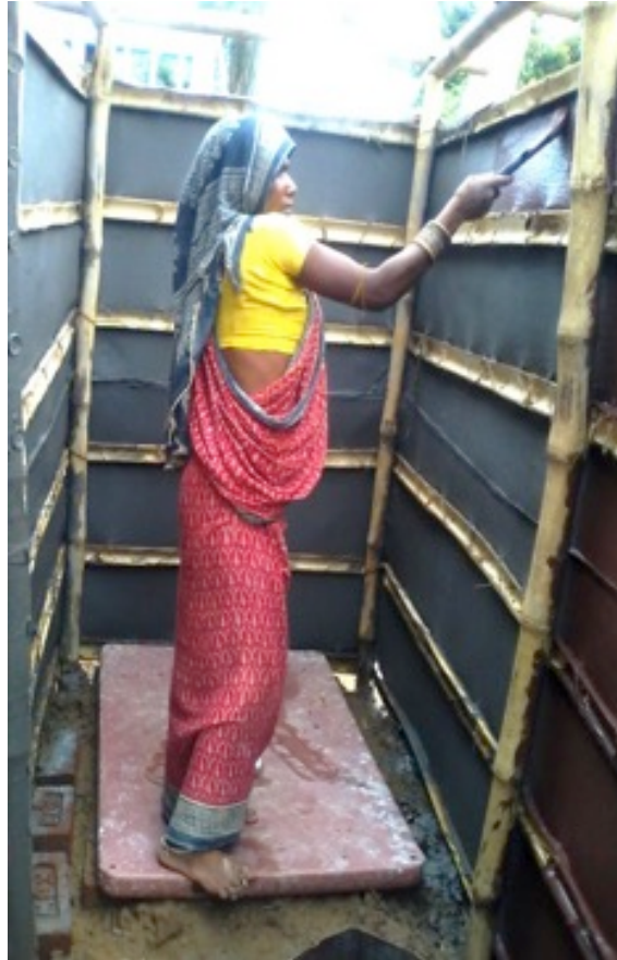
Image 6. 18: Construction of semi-permanent family latrines in Puri (Image Source: Agency A)
