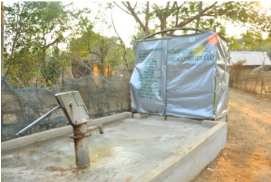
Image 6.17: Rehabilitated tube well and bathing facility (Image: Gopinathpur, 28-02-14)
