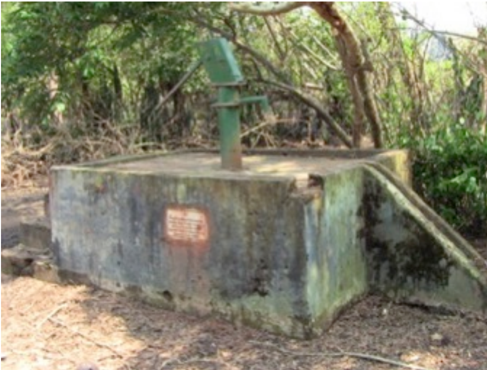
Image 6. 2: Pre-existing tube well built under Spanish Red Cross project as a preparedness measure after the 1999 super cyclone (Image: Piroshahi, 08-11-13)
