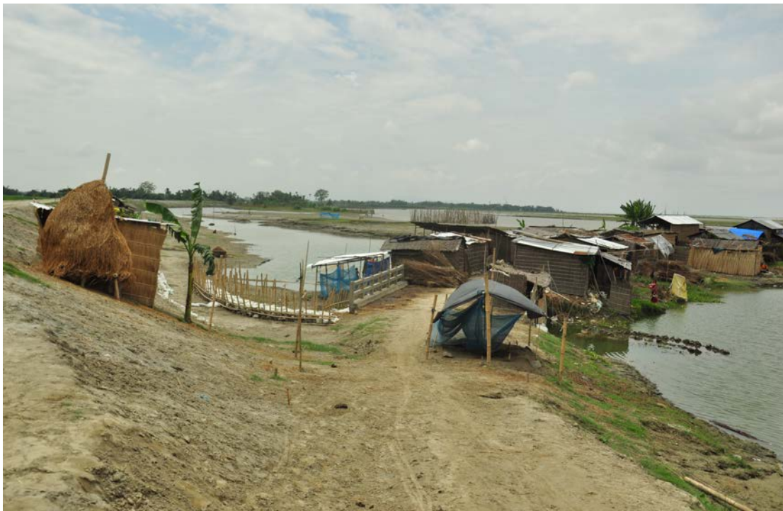
Image 5. 18: The above access road destroyed in 2013 floods (Image: Boramari, 04-09-13)
