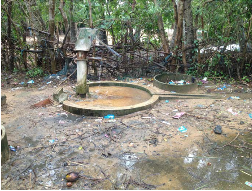
Image 6. 8: Debris near handpumps (Image: Gopinathpur, 24-10-13)
