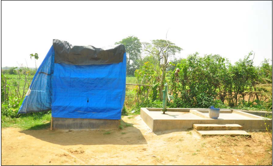
Image 6. 11: Sole communal hand pump and bathing facility for 28 households provided by Agency A (Image: Chadamankhana, 03-03-14)
