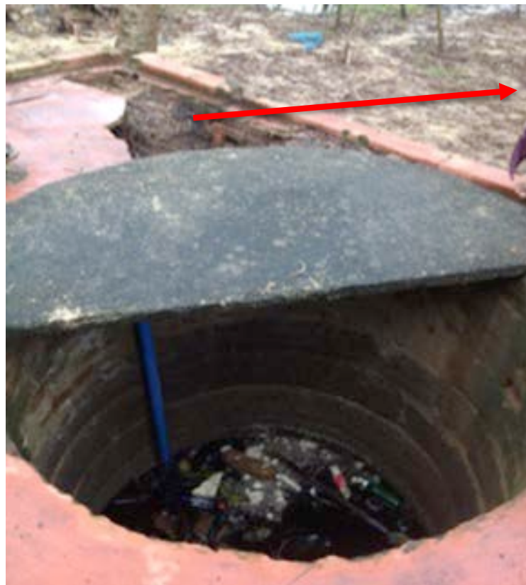
Image 6.7: Pre-existing protected open wells suffered structural damage during the cyclone
