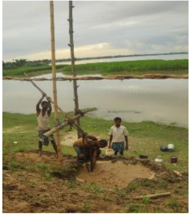
Image 5. 8: Installation of handpumps on the embankment (Image: Sonitpur, 13-07-12)
