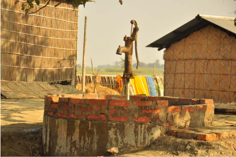
Image 5. 11: Newly installed hand pump on a raised platform (Image: Boramari, 09-01-13)
