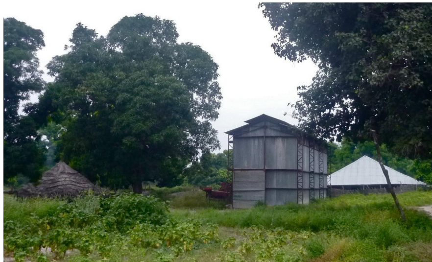
Fig.4.7 Colonial peanut depot, still in use. Payoungou.
