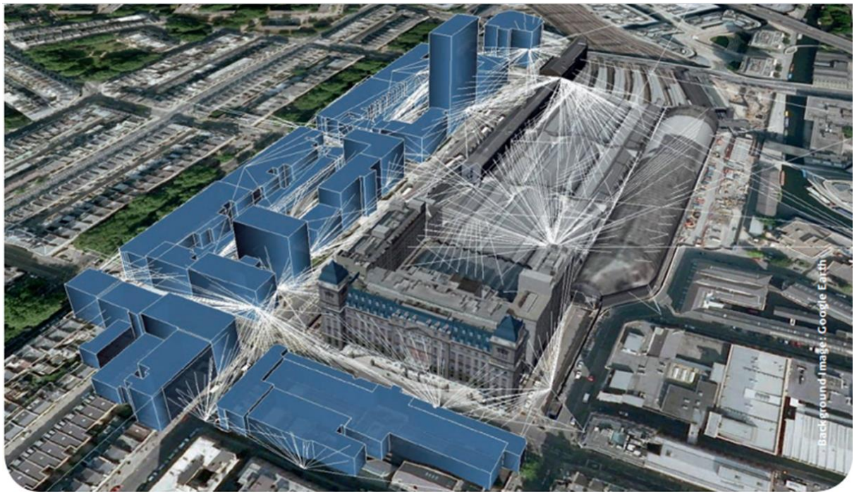
Figure 3.7: Example of large-scale automatic monitoring network on the CrossRail project including 52 total stations - image taken from Binder (2014)
