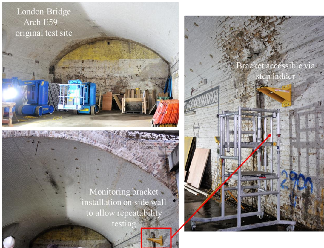
Figure 6.2: Images from original arch test site inspection
