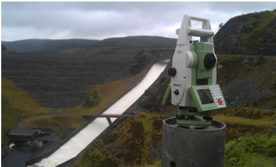
Figure 3.2: An example of a total station on a fixed pillar for deformation monitoring
