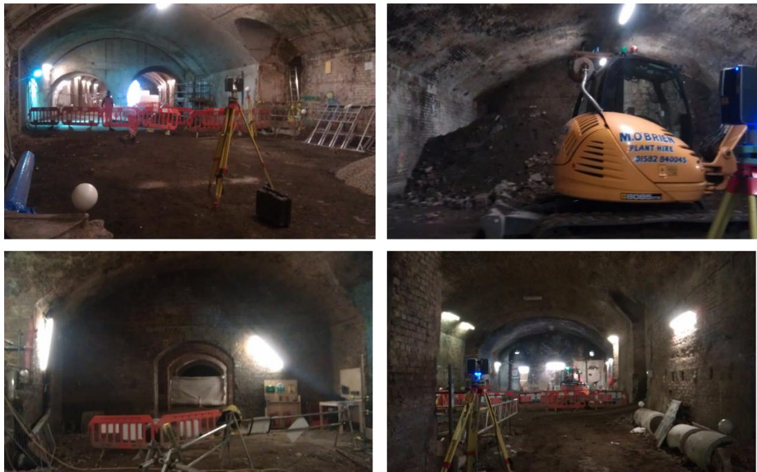
Figure 6.3 : Typical site conditions of arches during data capture
