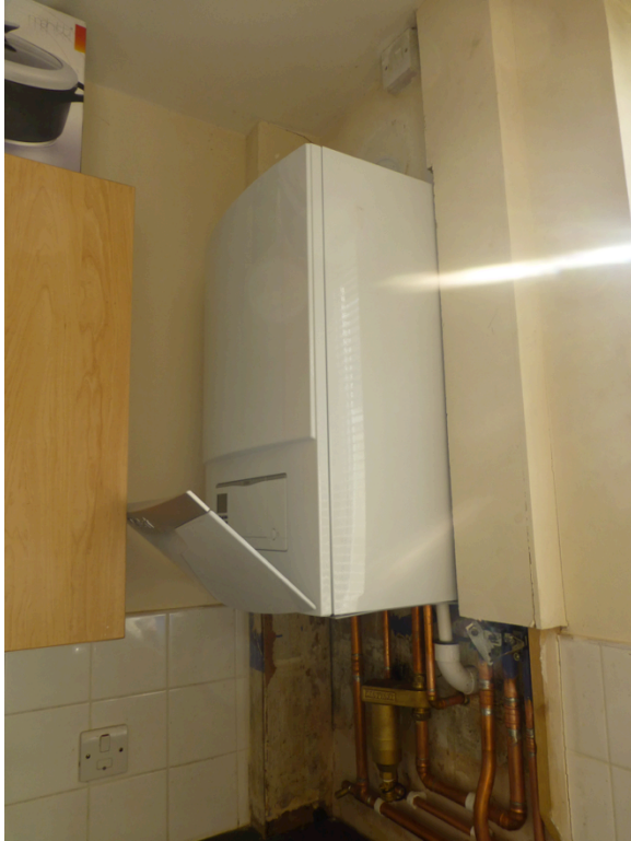
Figure 7.2 A user friendly installation?
