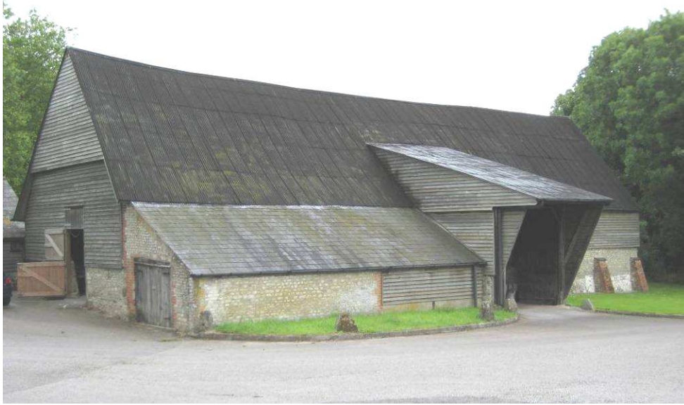
Figure 3: General view of the barn viewed looking north-west (photo Matt Hurford)
