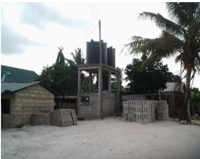
Image 1: Privately installed tanks with piped network to individual household in Tungi
