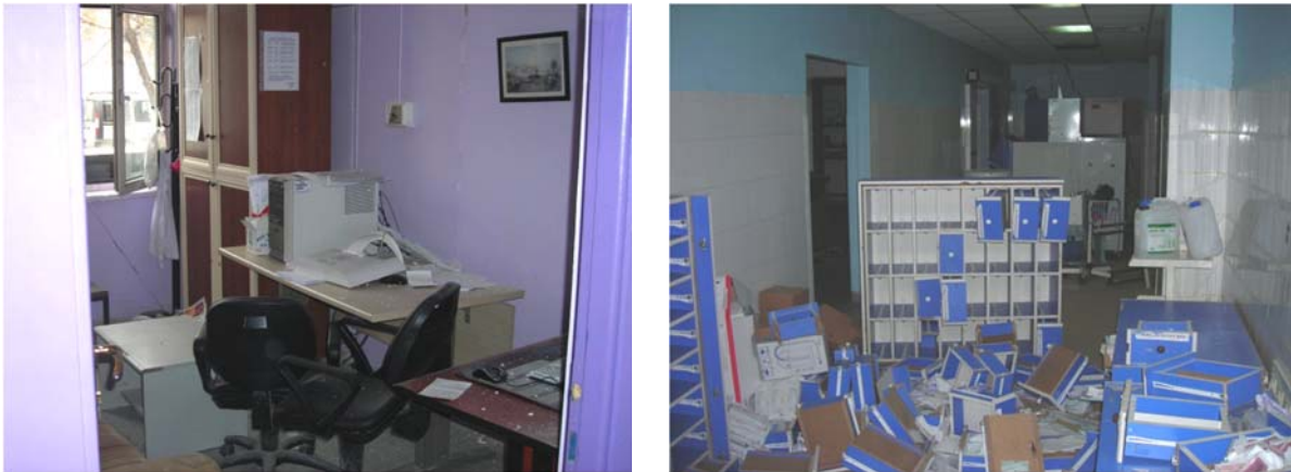
Figure 2. Damage to the building contents surveyed in the aftermath of the 2011 Van (Turkey) earthquake in the Yüzüncü Yil University – Faculty of Medicine Hospital.
