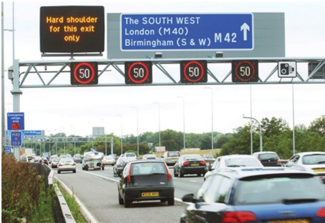
FIGURE 1.6: Operation of hard shoulder running on the M42 Motorway
