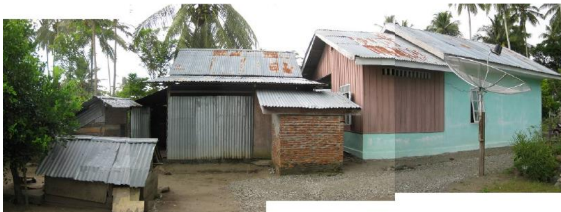
Figure 3: HFH's core home design (far right) in one community in Indonesia which incorporates the re-use of a timber transitional shelter as a kitchen (right) and later extensions using a combination of timber and other materials (centre and left).
