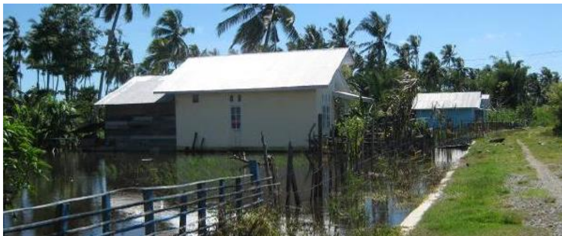
Figure 1: Flooded houses in Indonesia at the time of the assessment
