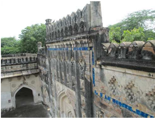
Figure 6.11 A close-up view of the band of turquoise coloured tiles employed on the wall-mosque.
