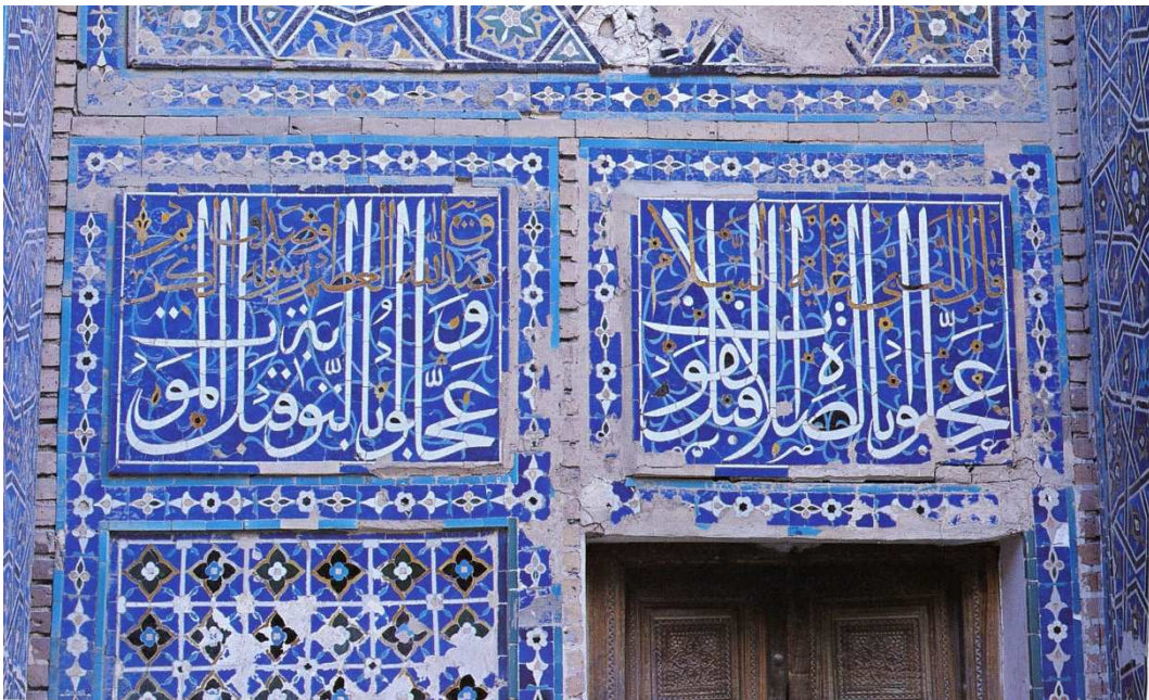
Figure 2.6 Techniques and typologies of tile-work employed by the Timurids on their buildings. (Top left) Glazed bricks laid in the banna'i technique on the northern facade of the mausoleum of Tuman Aqa (1404-1405 CE) in the Shah-i Zindah complex in Samarkand (from Soustiel and Porter 2003, p 139). (Top right) A haft rang polychrome glazed tile panel in the mausoleum of Amir Burunduq (c. 1390-1420 CE), also located in the same complex (from Soustiel and Porter 2003, p 130). (Bottom) Glazed tiles laid in the tile-mosaic technique, above and around the door of the prayer room in the complex of Tuman Aqa (1404-1405 CE) (from Soustiel and Porter 2003, p 136).
