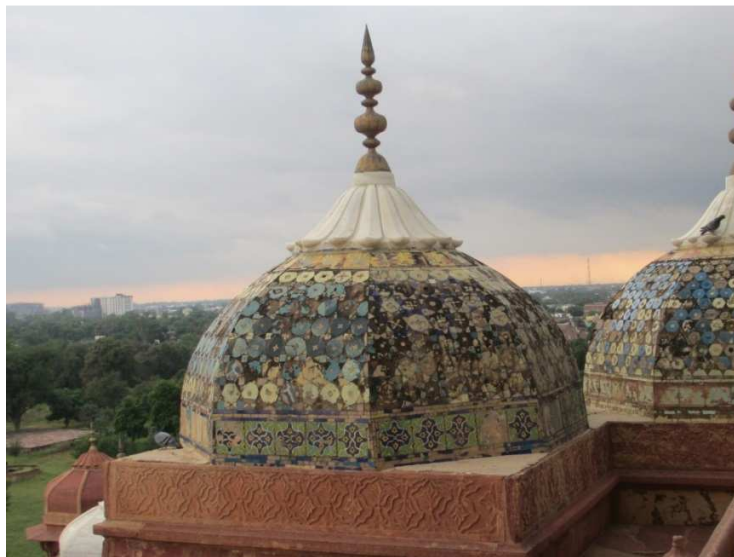
Figure 7.4 A general view of the tiling employed on a chhatri at the Tomb of Akbar. The unusual use of individual polychrome haft rang tiles in addition to monochrome tiles set in mosaic compositions is evidenced here.
