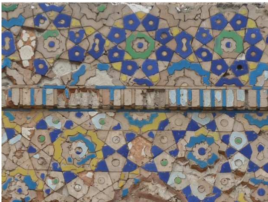
Figure 7.19 Detail of a portion of the tile-mosaic on the north facade. Note the apparent stage-wise loss of glazes on their separation from the bodies.
