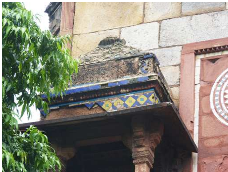
Figure 7.12 Detail of the tile-work on one of the jharokhas on the north gateway.
