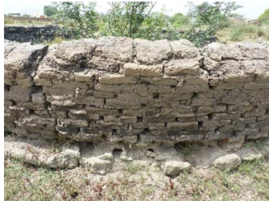
Figure 5.7 Close up of the exterior of the Akrabad furnace illustrating the use of sun-dried mud bricks for its construction.
