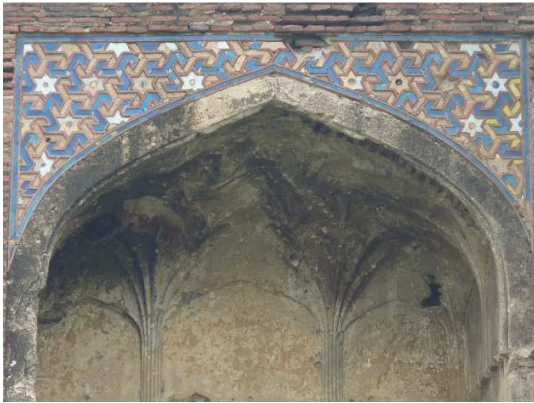
Figure 7.30 Tile-work on the spandrel of one of the smaller arches on the gateway. Note the use of unglazed bricks to separate individual tiles in the composition.
