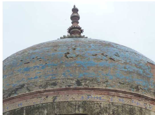
Figure 7.20 Close-up of the tile-work employed on the dome and drum. The dome carries tiles of a turquoise colour only, while the drum has a band of tiles of different colours laid in the mosaic fashion.
