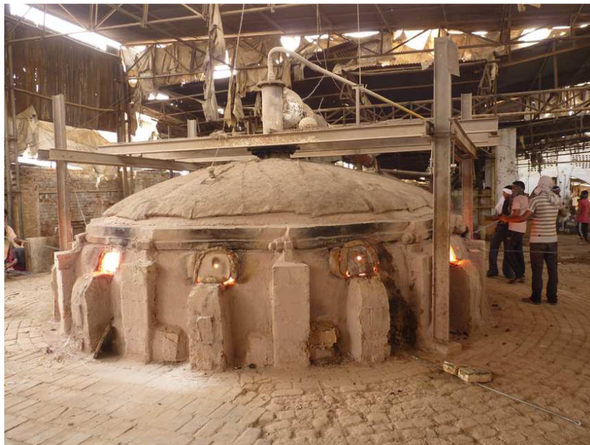
Figure 5.3 A modern gas-fired glass furnace in a factory at Firozabad.
