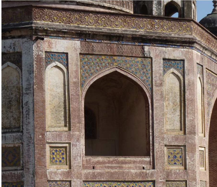
Figure 3.12 Tiled panels on the facade of the Tomb of Ustad (1612 CE) at Nakodar. The technique of application seen here, of tiles inset in geometric compositions of raised bricks, is a peculiarity of early seventeenth century tiling in the region, in the period of Jahangir.
