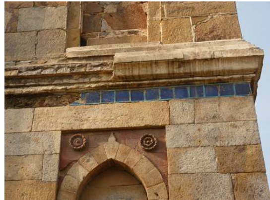
Figure 6.9 Detail of a band of dark-blue coloured tiles employed on the building, a colour rarity for Lodhi tile-work.
