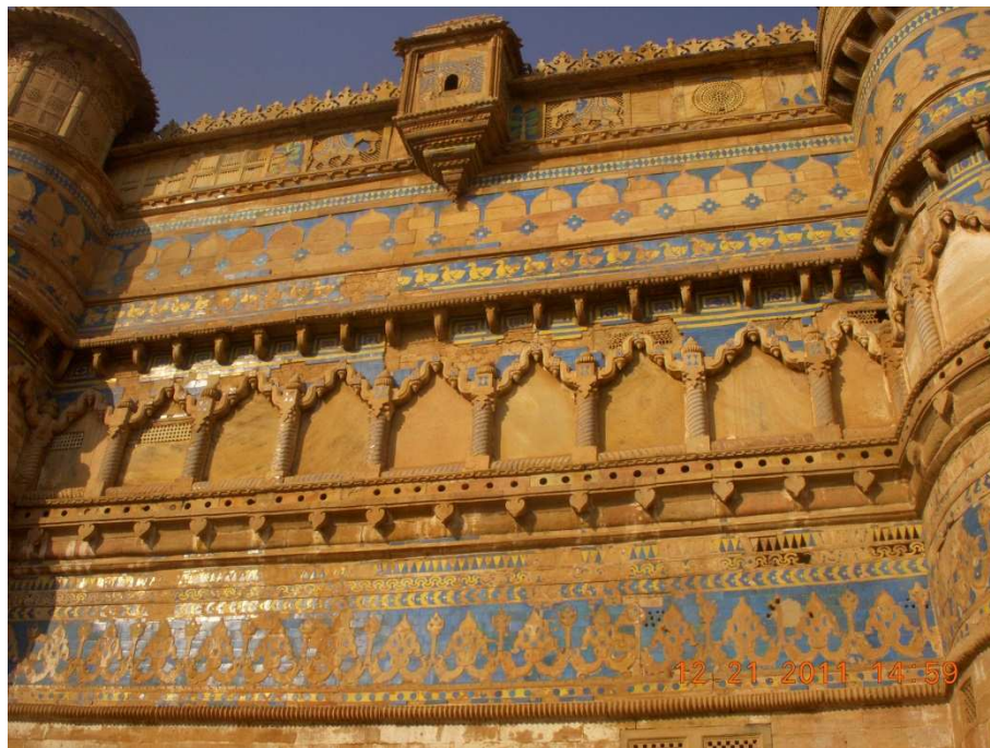
Figure 3.6 Glazed tile decoration on the exteriors of Man Singh Mahal (1489-1516 CE) in Gwalior Fort. The fort and building, a rare specimen of Hindu tiling for the period, was taken over by the Lodhis in 1518 CE.
