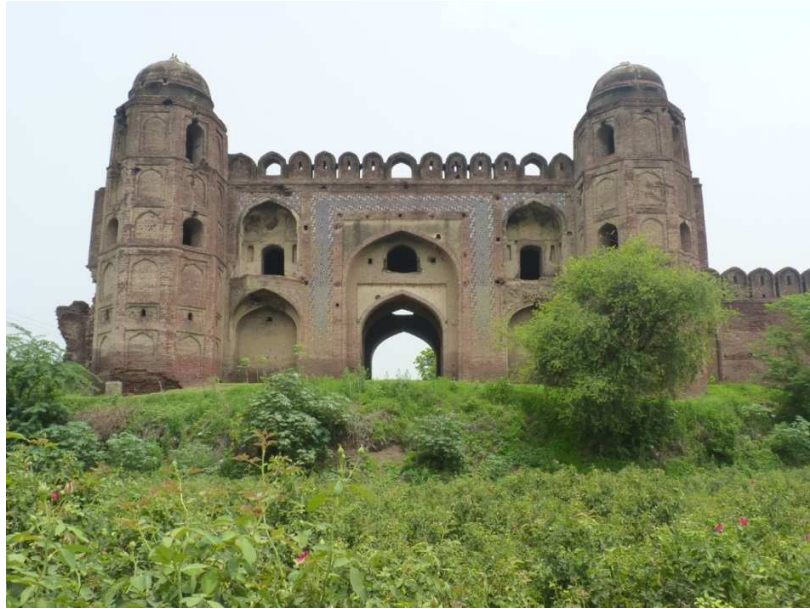
Figure 7.29 A general view of the southern gateway of Doraha Sarai.
