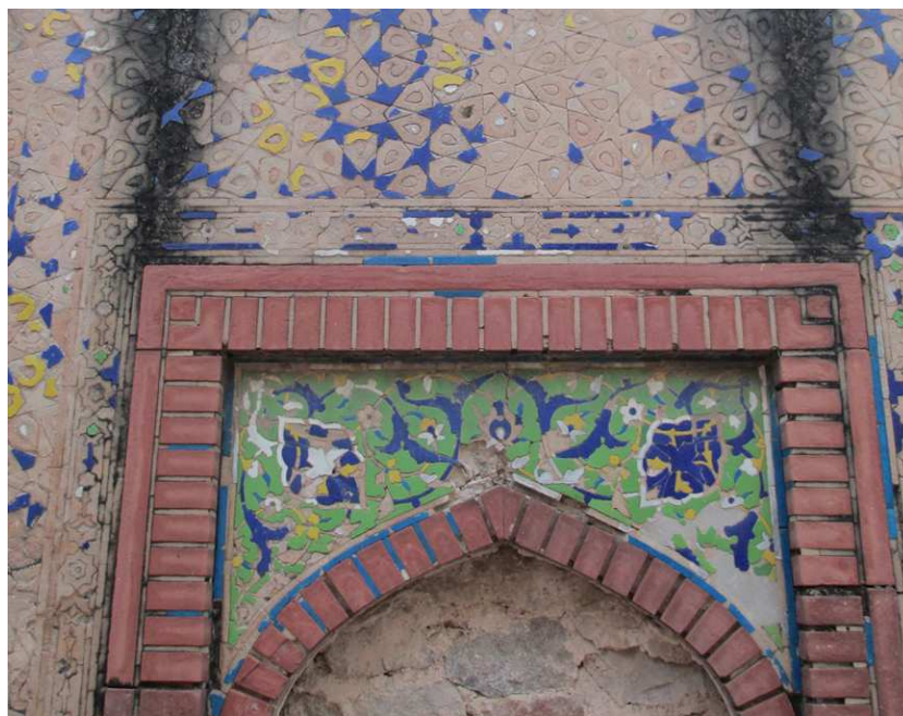
Figure 3.11. Detail of the tile-work employed on the wall-mosque at the Tomb of Atgah Khan (1566-1567 CE). The range of five colours and mosaic form of application seen here is typical of tile-work employed in Delhi in the sixteenth century during Akbar's rule.
