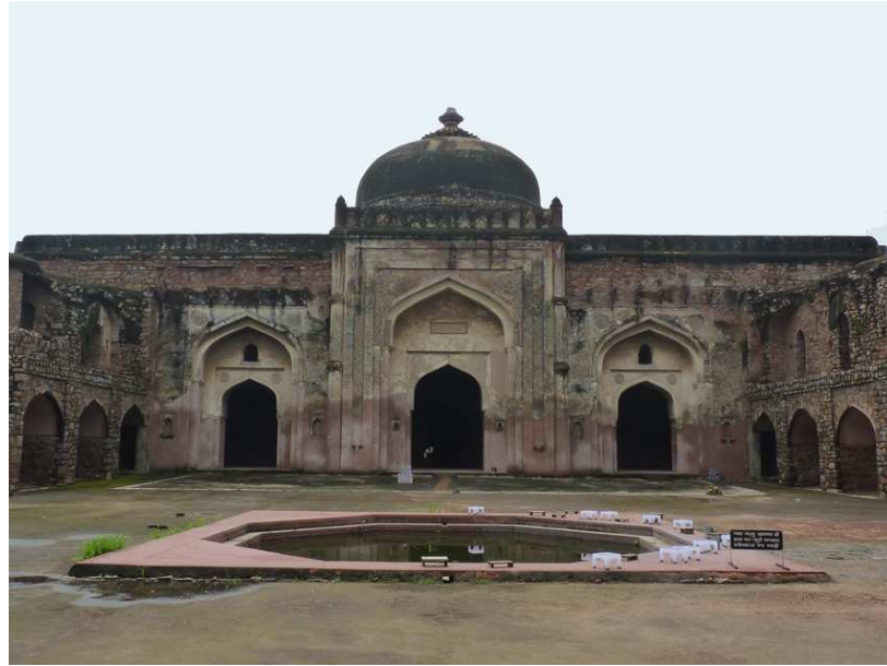
Figure 7.13 A general view of the mosque-structure in Khairul Manzil Masjid.
