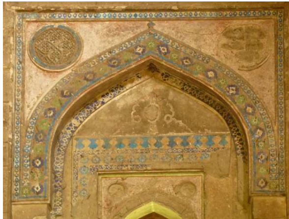
Figure 6.14 Detail of the tile-work in the interiors of the tomb, illustrating a relatively lavish use of tiles of turquoise, dark-blue, yellow, and green colours.
