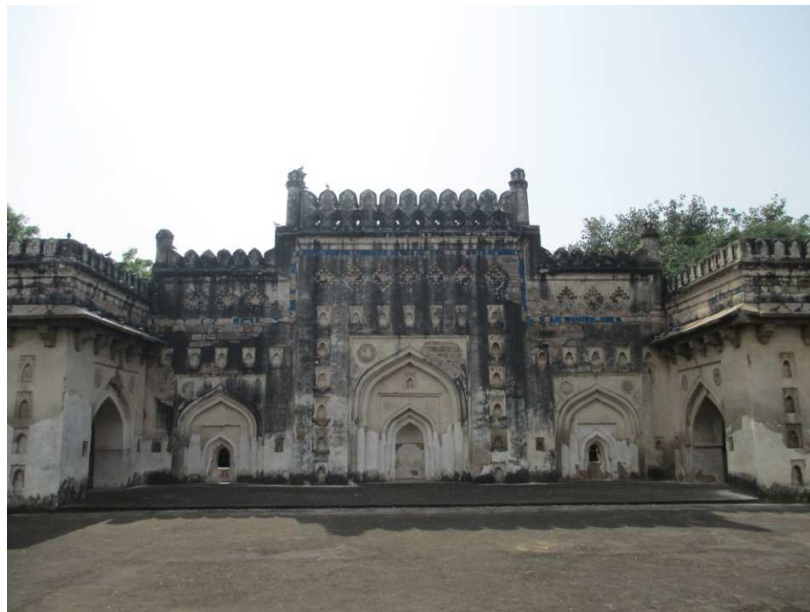
Figure 6.10 A general view of Madhi Masjid.
