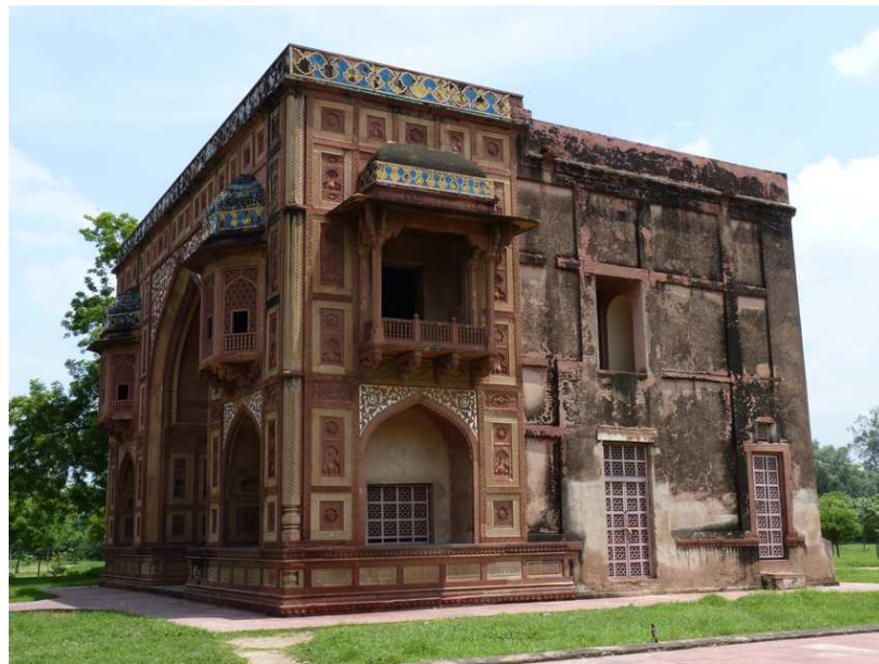
Figure 7.22 A general view of Kanch Mahal and its tile-work decoration.
