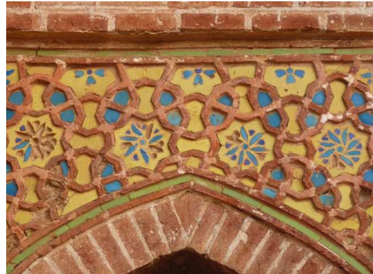
Figure 7.35 Tile-work on the spandrel of an arch. Note the floral patterns realised through the tile-in-tile inlay technique.
