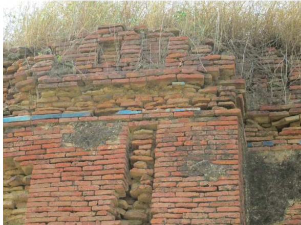
Figure 6.19 Detail illustrating the original use of glazed tiles in a band set between horizontally placed glazed bricks, the technique being the same as that used at the Bibi Taj-ka Maqbara.
