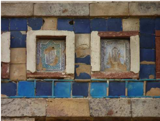
Figure 6.8 Detail of one of the friezes on the central projecting portions containing underglaze-painted blue-and-white tiles.
