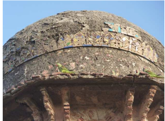
Figure 7.39 Close-up of the dome of a chhatri on the western gateway illustrating the use of tiles for its embellishment.
