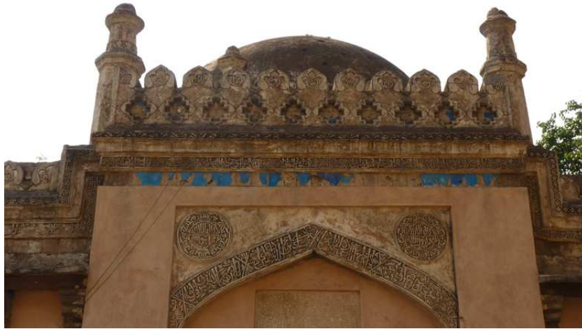
Figure 3.8 A band of turquoise coloured glazed tiles above the main portal of Nili Masjid (1505-1506 CE) in Delhi exemplifies the most common form of tiling employed by the Lodhis. The band of tiles in this case, and in many others, runs across the entire length of the front elevation of the building.
