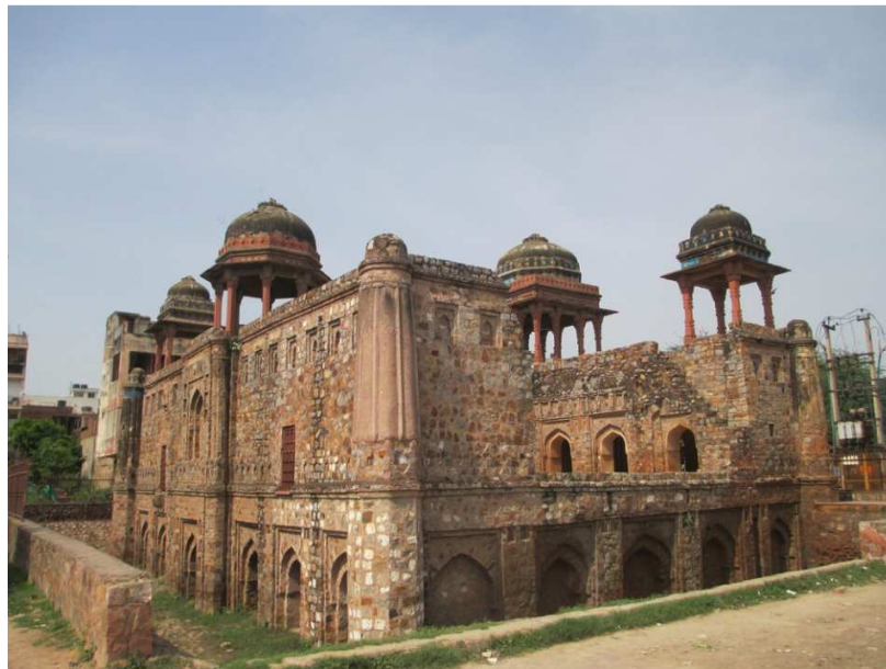
Figure 6.15 A general view of Jahaz Mahal.
