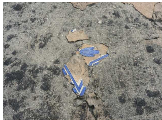
Figure 7.37 Fragment of an underglaze-painted tile employed on a dome. The grey coloured material on its sides is cement mortar from repair work.
