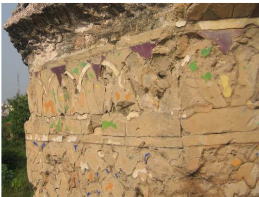
Figure 7.36 Detail of the tile-mosaic employed on one of the corner domes. The use of purple and orange coloured tiles can be determined here, in addition to the common repertory of five colours.
