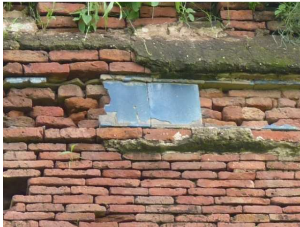
Figure 6.17 Detail illustrating the use of glazed tiles in conjunction with glazed bricks, the latter being the ones laid horizontally.
