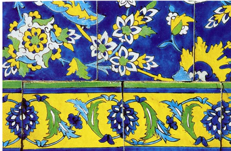
Figure 2.9 A panel and border of polychrome haft rang tiles on the Shah Mosque (c. 1611-1627 CE) at Isfahan, Iran. Such tiles were typically preferred over the tile-mosaic in Safavid tiling of the early seventeenth century, the shades of colour employed on these tiles also typical of this time (from Degeorge and Porter 2002, p. 148).
