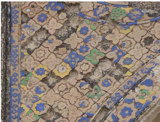
Figure 7.14 Detail of the tile-work affixed in mosaic compositions on the exteriors of the central arch of the mosque-structure.
