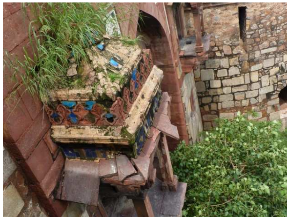
Figure 7.9 Detail of the tile-work on one of the jharokhas on the external facade of the gateway.
