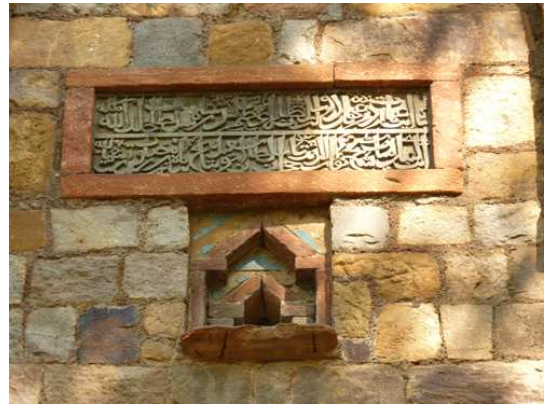
Figure 6.6 Detail of the tile-work below the inscription on the western wall.
