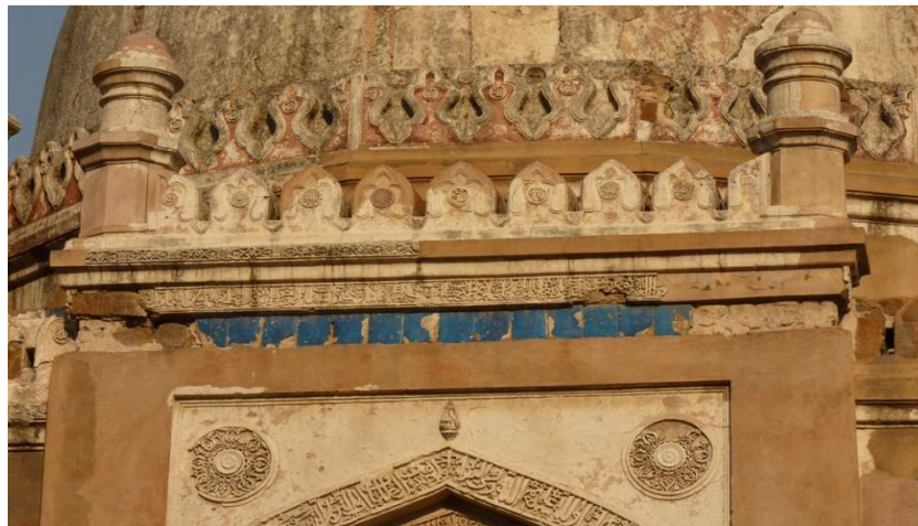
Figure 3.7 A band of blue coloured tiles on the tomb called Chhote Khan-ka Gumbad (early sixteenth century) at Delhi, illustrates the restraint exhibited in tiling during Lodhi times.
