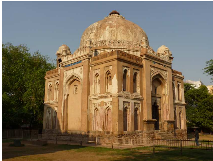
Figure 6.2 The restraint that marks Lodhi tile-work, and its common form of application, as a single row or band, are both well-illustrated in the case of tiling on Chhote Khan-ka Gumbad seen above.
