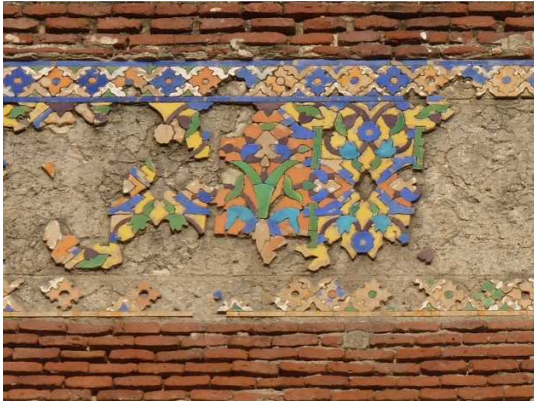
Figure 7.38 Detail of a portion of the tile-work on the western gateway. The use of seven distinct glaze colours can be evidenced in the mosaic composition depicted here.
