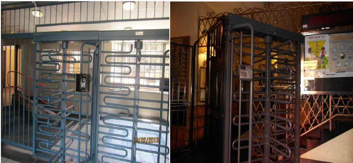
Image 7: Entrance to a communal housing building, Jeppestown (photograph by the author)
