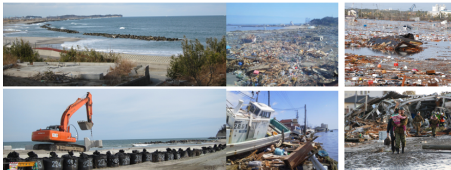
Figure 6.2: Soma City Devastation and Temporary Tsunami Barrier
