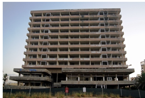
Fig 7.17. Graffiti (much of it erased) on the first floor of this building reads ‘Fotoğraf ve Film Çekmek Yasaktır’ (Photography and Film are Forbidden). Photograph author’s own
