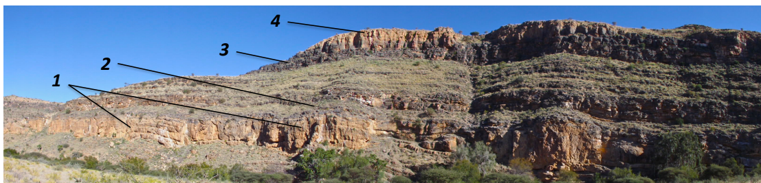
Figure 1.22: Photo of typical section of OS1 and OS2 at Zebra River. Vertical scale is 160 m 1 - Laterally extensive orangy-brown microbial biostrome containing individual reef mounds, separated by inter-reef shales and marls. 2 - Termination of reef growth and a sequence of grainstones and subordinate shales 3 - Grainstone horizons become more closely spaced towards top of OS2 4 - A dolomitised Metazoan-packstone marking the Omkyk to Hoogland member transition
