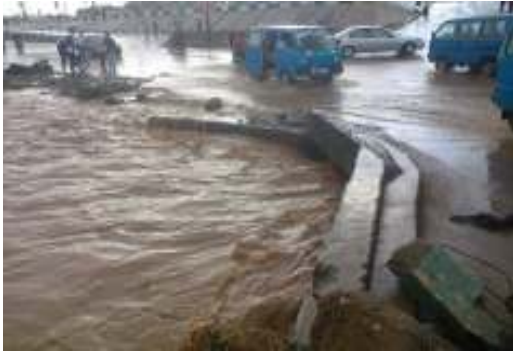
Figures 3 (a) and (b) Undersized Rasco culvert being submerged during storms of October/November, 2013
