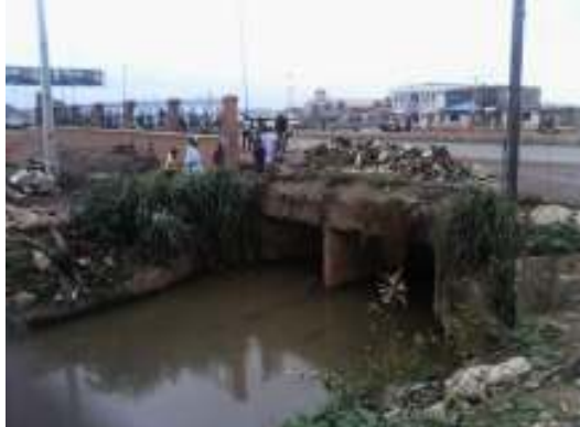
Figure 4 Undersized culverts at (a) Alakewudo (Sawmill) (b) Rasco Hall
