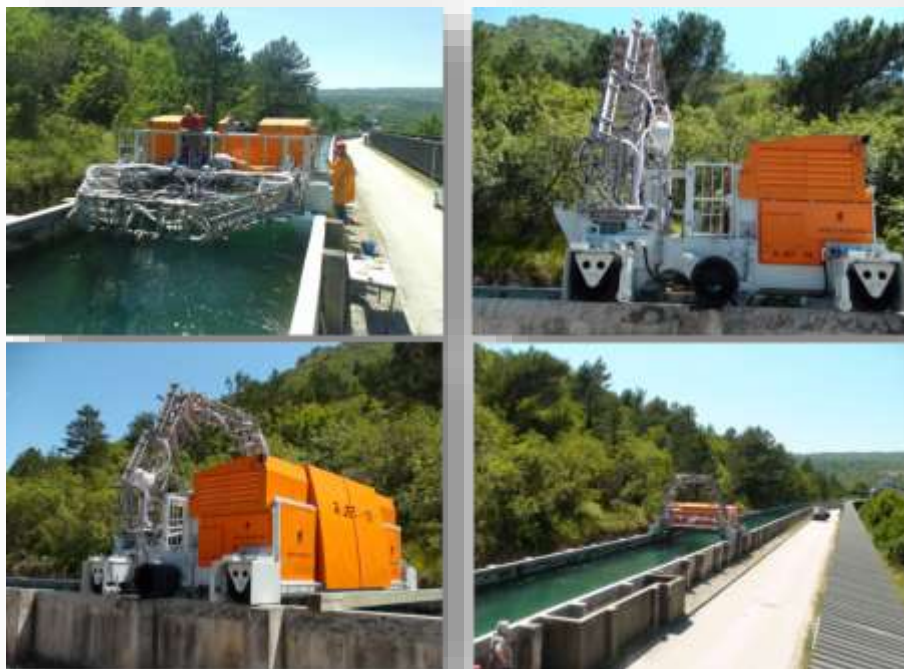
Figure 1 R JET 111 design, construction and implementation at the TE Plomin, Croatia
