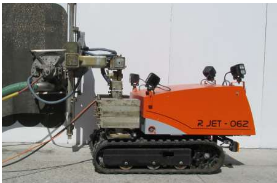
Figure 6. Hydrodynamic paint removal treatment applied to the concrete wall surface.
