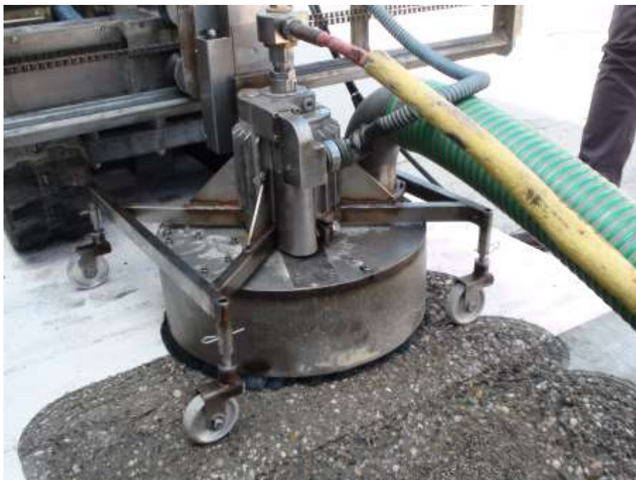
Figure 5. Hydrodynamic treatment applied to the concrete floor surface.
