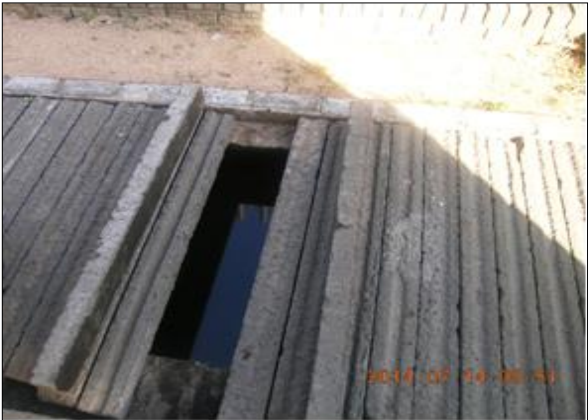
Figure 14: Grit chamber at one commercial carwash facility (By author)
