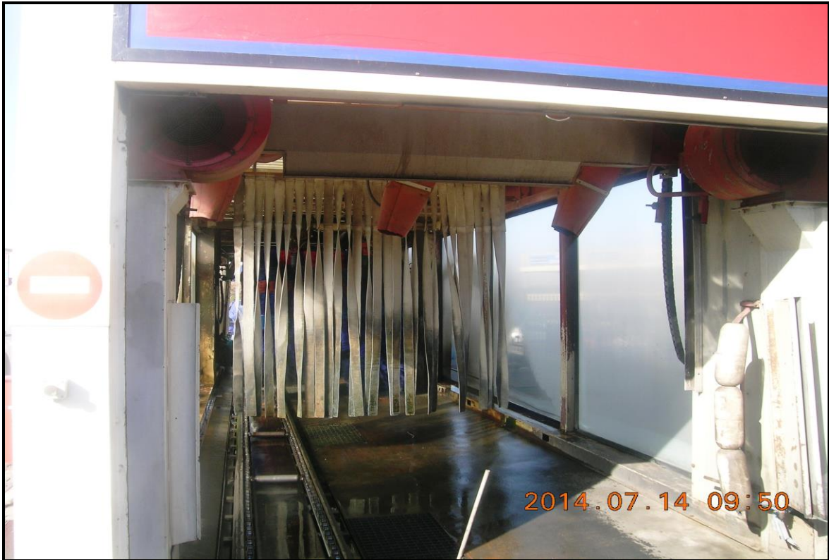
Figure 2: Conveyor car wash (by author)
