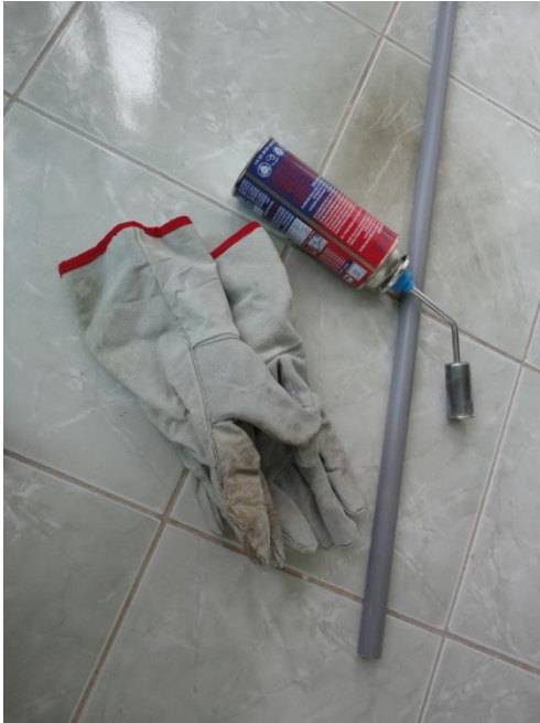
Figure 5.7 PVC pipe ready to be heated.
