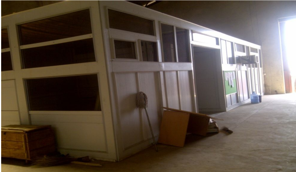
Figure 5: a complete assembled PVC structure used as an office in IBP industry, Idu yard, Abuja.
