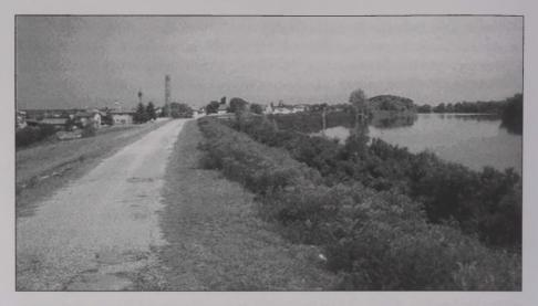
Figure 4: Po river embankment: normal flood level is higher than ground level. The village in the picture is next to the embankment, increasing vulnerability.
