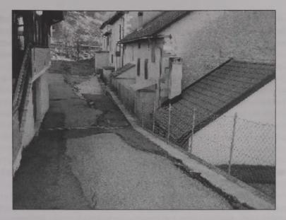
Figure 3: Lamosano, damages caused by local lowering movements in a restaurant parking. The restaurant is closed but the owners are still living there, even if the building shows serious damage.
