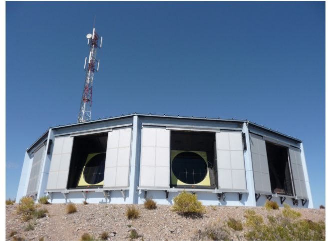
Fig. 6. FD building at Los Leones during the day. Behind the building is a communication tower. This photo was taken during daytime when shutters were opened because of maintenance.
