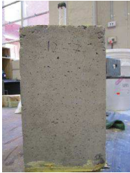
(a) Bar slippage. Fig. 2 Failure modes
