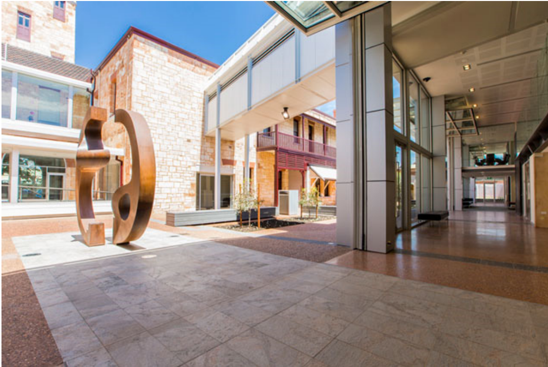
Figure 2: Kalgoorlie Court Complex: The new and older heritage buildings of the Kalgoorlie Court Complex were integrated through the installation of a series of courtyards which can be enclosed with glass panels. The panels can be drawn back to allowing the internal and external areas to have a seamless connection. Aboriginal people from rural and remote areas (regions serviced by the courthouse) generally have a preference to waiting in outdoor spaces and have sightlines to watch other people. The courtyards can be used as external waiting areas and people can stay in contact with court proceedings while being outside. The areas are installed with sculptures completed by Aboriginal artists from the region to enhance Aboriginal 'ownership' of the courthouse and to establish the courthouse as an Aboriginal 'place'.
