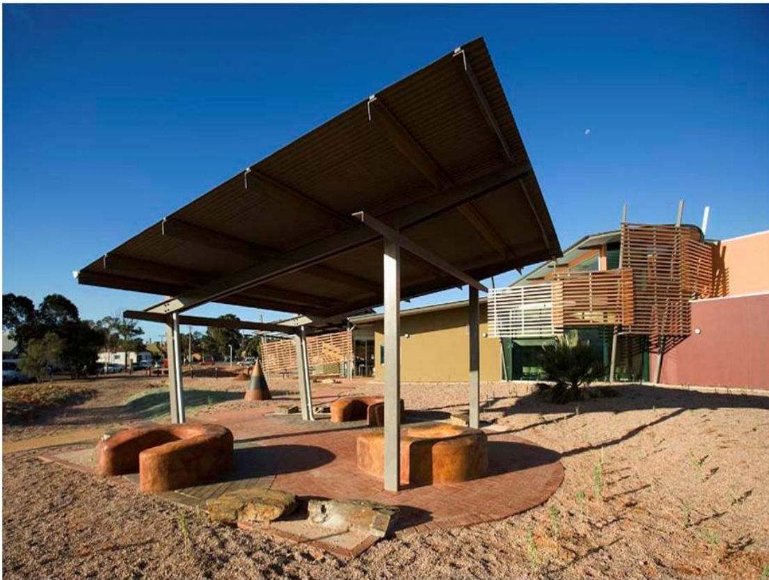
Figure 1: Port Augusta Court Complex: The courthouse is designed with a covered exterior area. The area was sited to provide sightlines to the approach and entrance of the building, the internal public waiting area and the culturally significant Flinders Ranges in the distance. It has also been positioned taking account of prevailing winds and sun patterns, as feeling the wind and sun on one's face is important to feelings of wellbeing for Aboriginal people from Desert regions. The design of the seats replicate figures used in Western Desert Art to show a person sitting. The seating was located as shown to allow Aboriginal people to sit in small groups and avoid direct eye contact with others as is the customary behavior. The external area has technology fitted to allow it to be used as an external court area. To date, it has not however, been used for this purpose.
