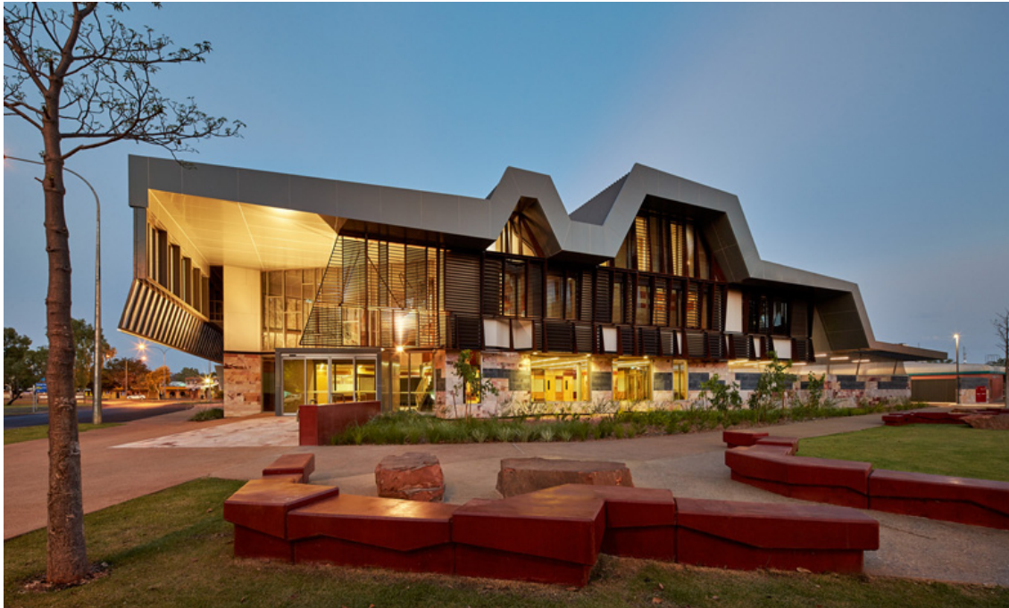
Figure 3: Kununurra Court Complex: The form of double storey building echoes the shapes of significant nearby landforms (i.e. Kelly's Knob and Hidden Valley) to provide a physical and figurative connection of the courthouse to 'Country.' An extensive use of glass paneling has been employed to allow Indigenous users to maintain connections with the external environment through short and long range sightlines. Various external waiting areas have been provided for Aboriginal people to allow them to spend time outside in informal gatherings.
