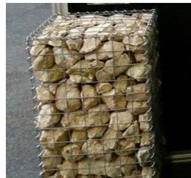
Figure 11 Trial Gabion Wall Construction
