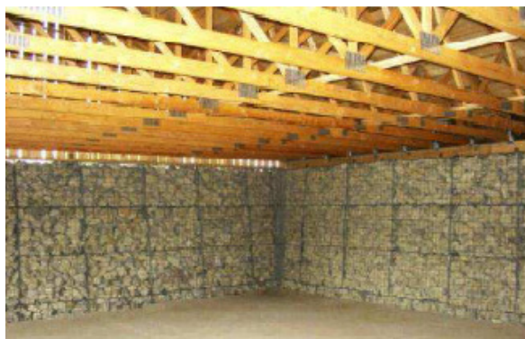
Figure 1 Walls of the Boat House ( HY-TEN Gabion Solutions, n.d. )
