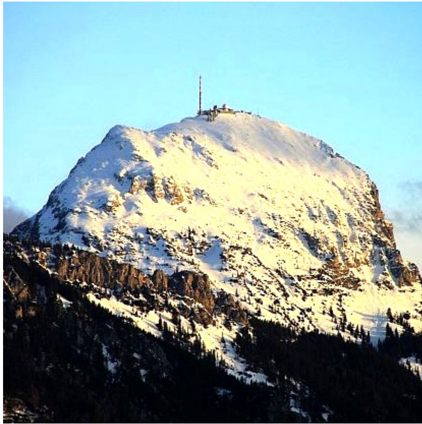
Figure 2.5: Image of the summit of mount Wendelstein, showing the radio antenna and 8.5 m dome of the observatory to the right.
