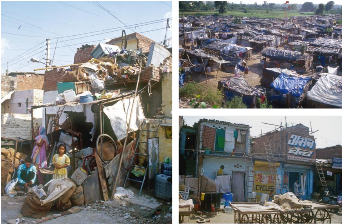
Figure 2-7: Different types of informal housing in Delhi, India (Photographs: S. Smollich, October 2005).
