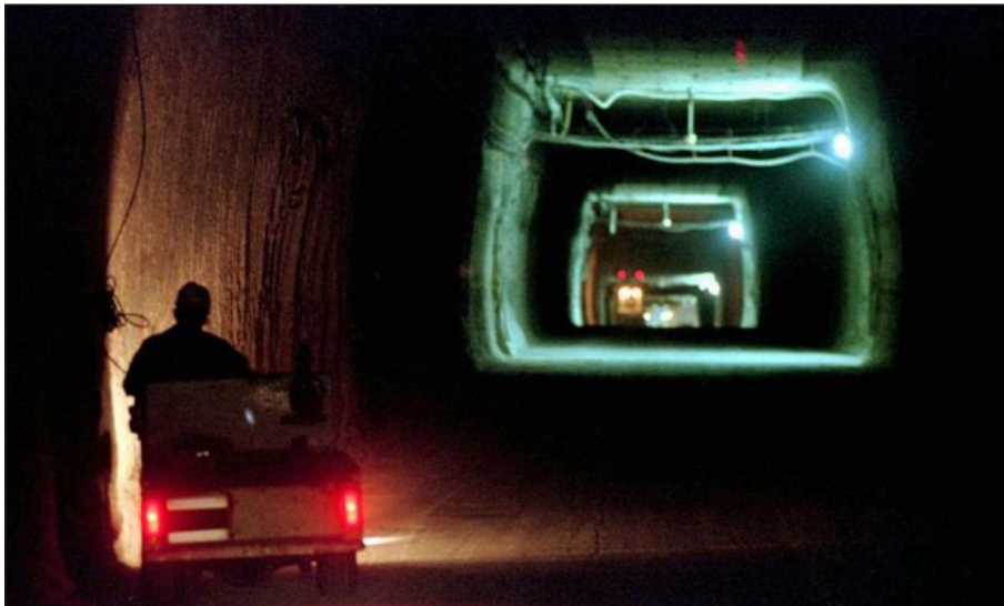
Construction of the Waste Isolation Pilot Plant in New Mexico, an underground nuclear waste dump. Photograph: Eric Draper / AP.
