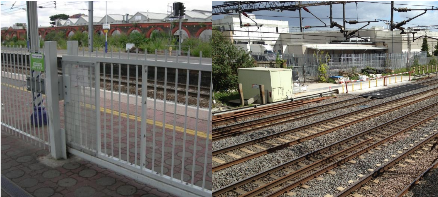
Figures 2a and 2b Photographs showing where a platform serving a fast line has been fenced off in an earlier intervention and where faster lines do not run close to platforms
