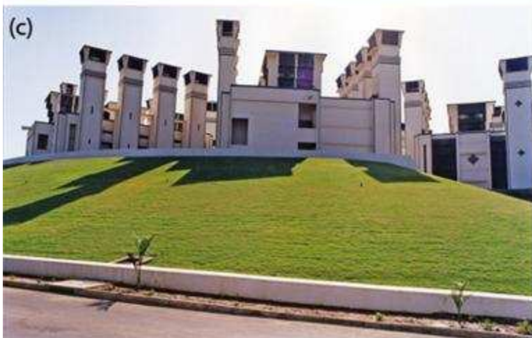
Fig. 9. Windcatchers in contemporary buildings: (a) Springs Preserve building in Las Vegas, USA; (b) Zion National Park Visitors Center in Utah, USA; (c) Torrent Research Center Building in Ahmedabad, India [65], [75] and [95].
