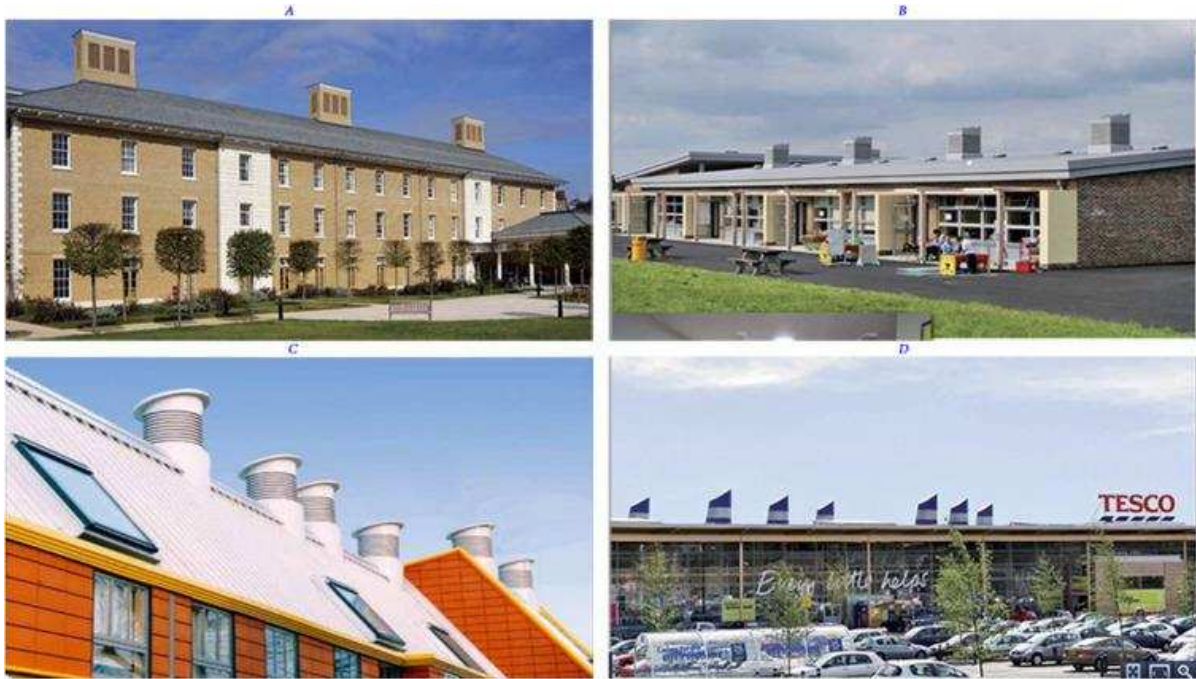
Fig. 7. Different Monodraught windcatchers in the UK: (A) Royal Chelsea hospital, London; (B) Seaside School, Lancing; (C) Addey and Stanhope school Deptford; (D) Tesco Eco-store Cheetham Hill [35].
