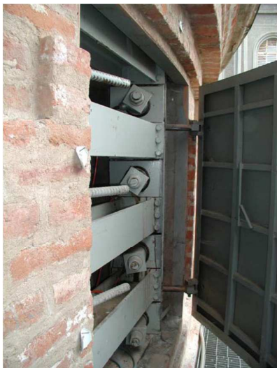
Figure 4. (a) Tie-bar ends equipped with load cells and (b) tie-bars end with the anchorage system.
