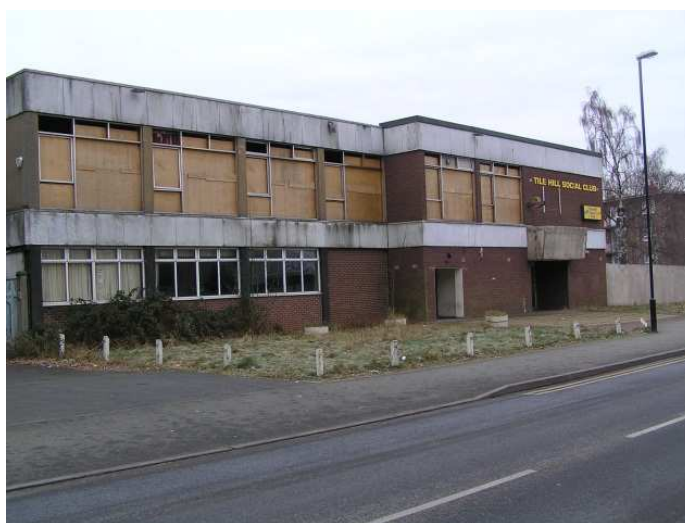
Plate 10: The Tile Hill social club closed down and sold out with boarded windows has been vandalised by the local youth (February 2012).
