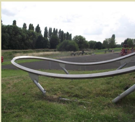
Figure 7: Broken play equipment at Babbs Mill
