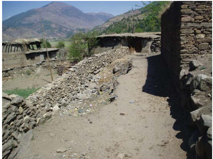
Picture 6: Incomplete segment of road/track, Kartikswami
