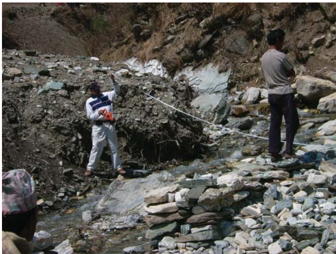
Picture 3: Measurement of canal repair works
