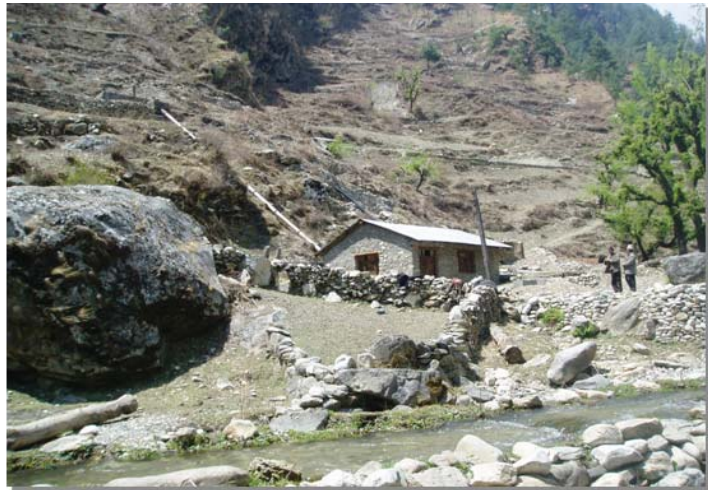
Picture 2: Power house, Patmara micro-hydro scheme
