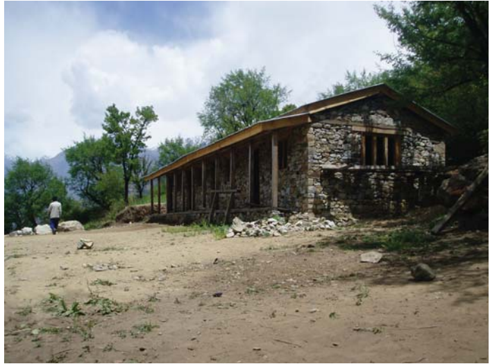
Picture 11: Newly built school and playground, Dandafaya
