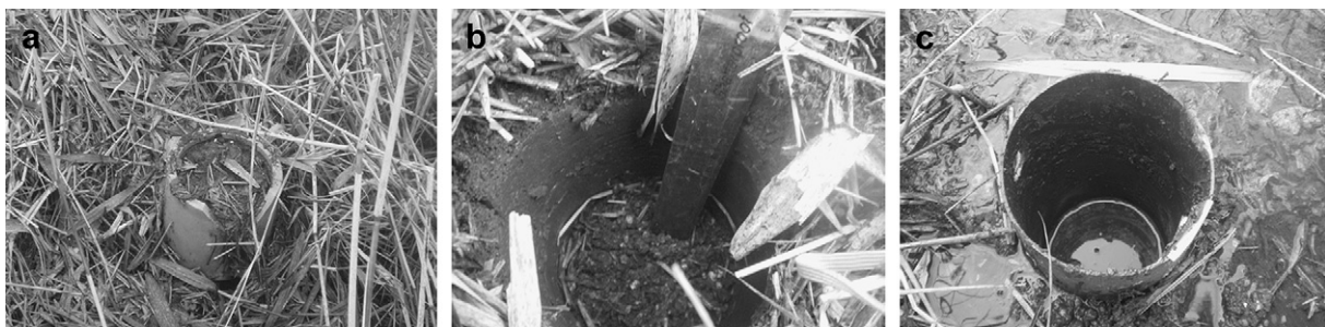
Fig. 2 – Photographs detailing the more prominent findings at the site, including a) Completely clogged inlet distributors, b) Surface sludge layers up to 200 mm thick at the inlet, c) two water levels at certain points in the system, representing disconnected overland and sub-surface flows.
