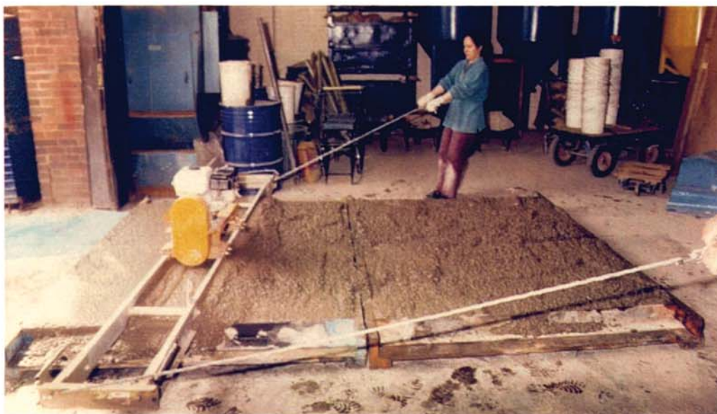
Plate 9.6 Screeding operations of ready mix concrete specimens
