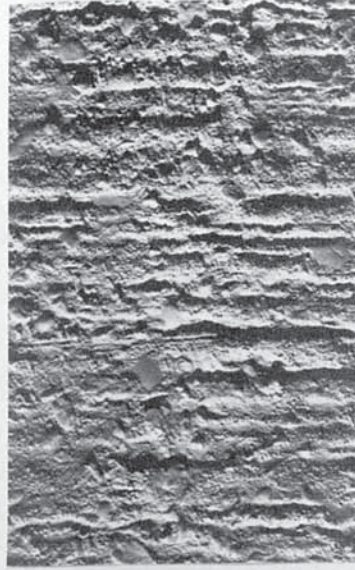
( 4 ) LATERAL BRUSHED CONCRETE
