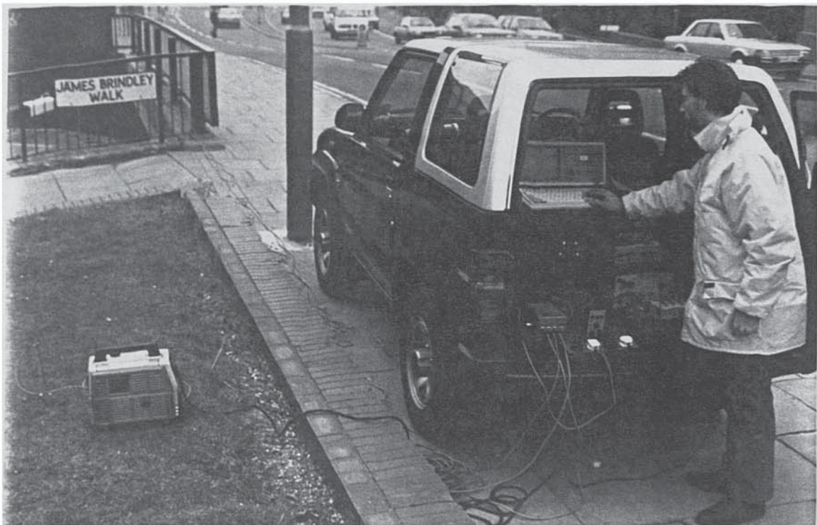
Figure 5.4 Acquiring site vibration data from one impact event
