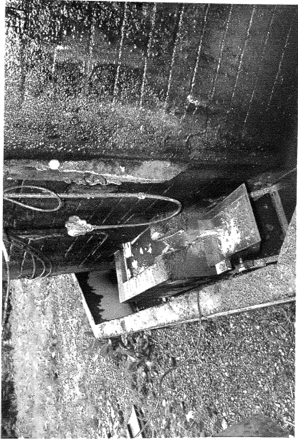
Plate 4.1.3 Primary filter effluent drain, sump and tipping trough used in flow recording. Showing Foster Cambridge temperature probe positioned in filter wall.
