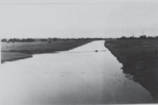
E. South Drain, Wessex Drainage dyke
