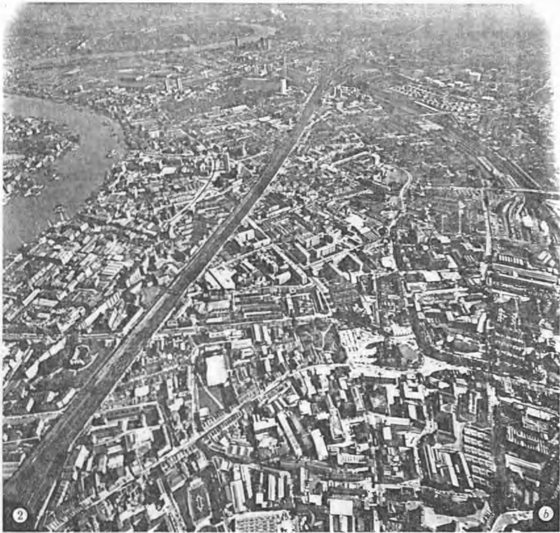
FIGURE 2 ( b ). Bermondsey and Isle of Dogs (SV 997). A high proportion of the total area has roof- and paved-cover and artificial surface drainage. Old buildings, probably with shallow foundations and small basements in Flood Plain gravel, predominate with some multi-storey blocks, probably with deep-piled foundations. The variable river-wall construction of the commercial waterfront and the large area occupied by the docks is well illustrated. The railway viaduct is a dominant feature, but probably has a shallow foundation and does not cut off the gravel stratum.
