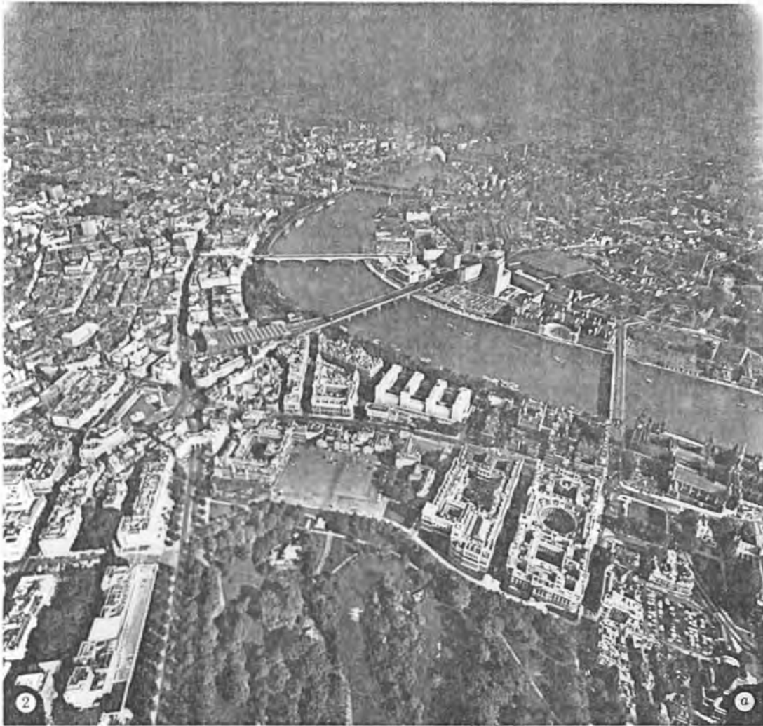
FIGURE 2. Oblique aerial photographs illustrating typical building and structures in the lower Thames Flood Plain. (Courtesy Aerofilms Ltd). (a) Kings Reach - Westminster - Waterloo (SV 10120). The narrow strip of Flood Plain on the north bank in the Central London area and the ground slope associated with its boundary is shown. The foreground includes the artificial lake in St James's Park and the complex of historic buildings in Westminster, whose original foundations and basements in general are probably shallow and thus potentially affected by changes in groundwater conditions. The modern developments on the south bank have pile foundations and extensive deep basements and subways which must interrupt the continuity of the Flood Plain strata. Much of the river wall in this area is relatively modern and has a deep foundation, nearly, or completely, cutting off the gravel stratum.
