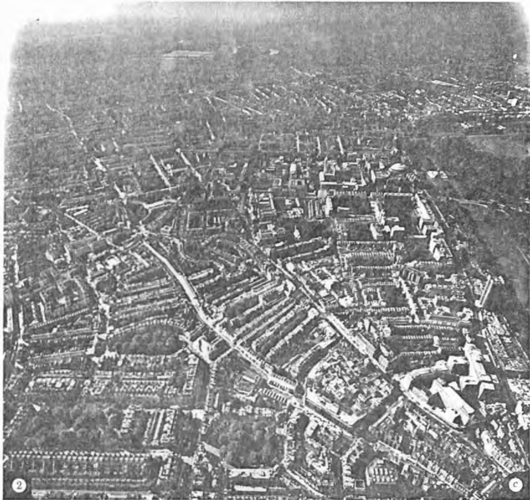
FIGURE 2 (c). Kensington area (SV 1009). A significantly higher proportion of open space than in (b). Dominantly terraced houses probably with shallow foundations and invariably with small basements in the Flood Plain gravel: increasing size of building is probably accompanied by increasing depth of basement, but shallow foundations were probably still employed.
