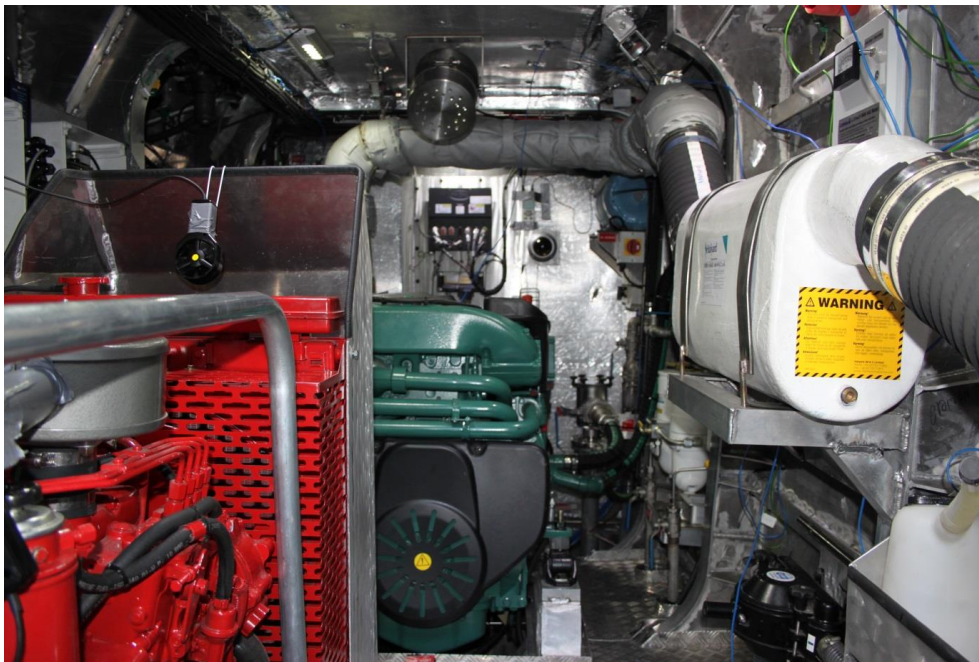
Fig. 1. Photograph of engine room showing the engine (green) and Genset (red).
