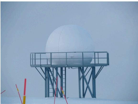
Figure 2. Protective dome housing the radar transponder based on Svalbard.
