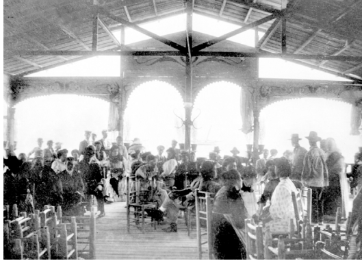
Figure 5: Cradle trusses and joggle-posts inside the bathing resort in Torrevieja. Photo Collection, image on disc 3-7 and 3-3.
