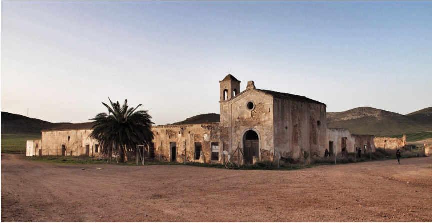
Figure 1: Present condition of the Cortijo del Fraile (2015) (photo by the authors).
