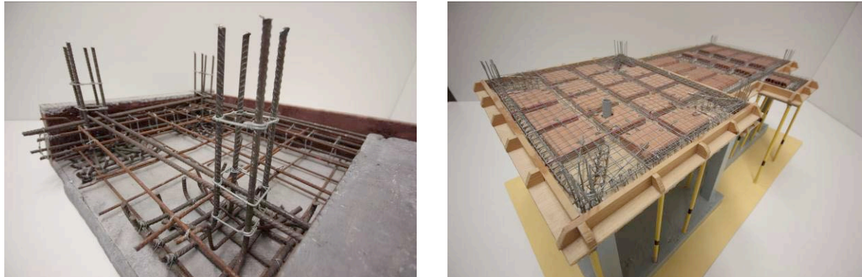
Figure 1. Mock-ups for the exhibition. Left image: mock-up of foundations footings. Right image: mock-up of a reticular forging.
