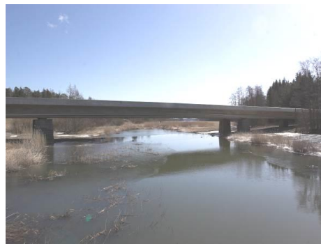
Fig. 19. Same area after bridge construction.
