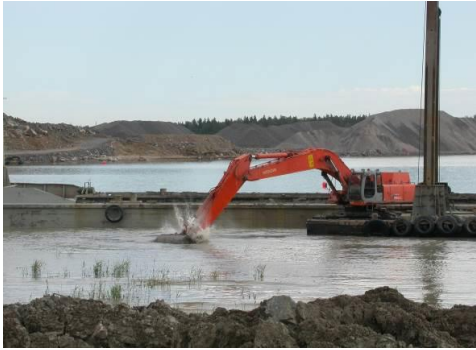
Fig. 2. Dredging of mud and clay at harbour site.
