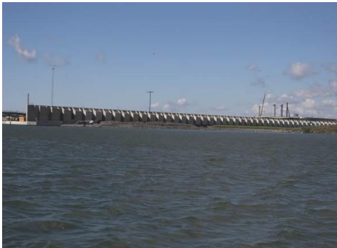
Fig. 4. A 1.3 kilometre long wall was built at the edge of the harbour to reduce noise and visual disturbance at Natura 2000 area.
