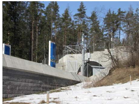
Fig. 17. Railway tunnel at Labbacka.
