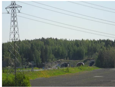
Fig. 11. Road and railway crossess Österängen and tunnels go through Labbacka forest.
